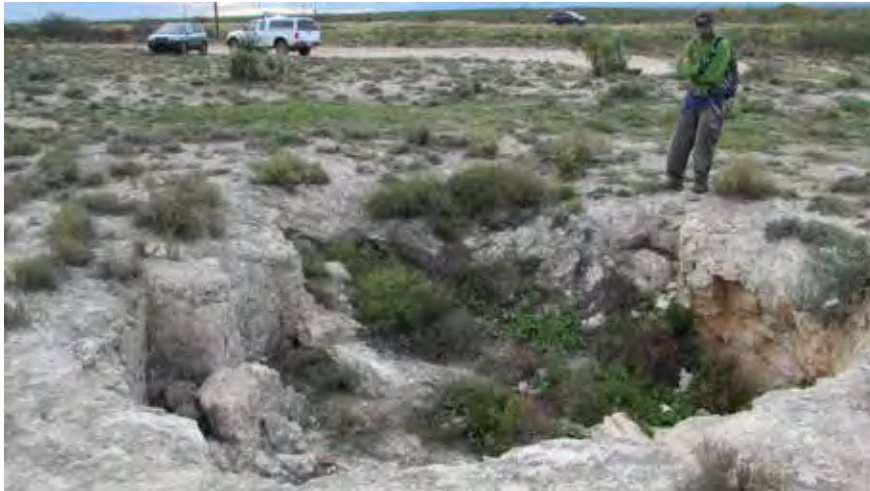
Figure A15. Station 12.0E sinkhole A.
