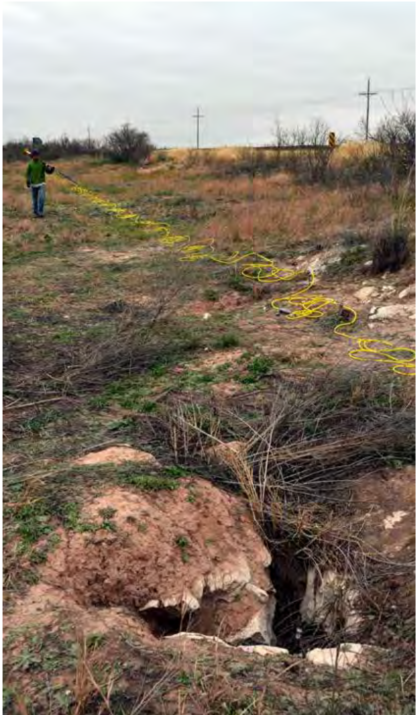
Figure A7. Station 8.6W sinkhole and ER cable.
