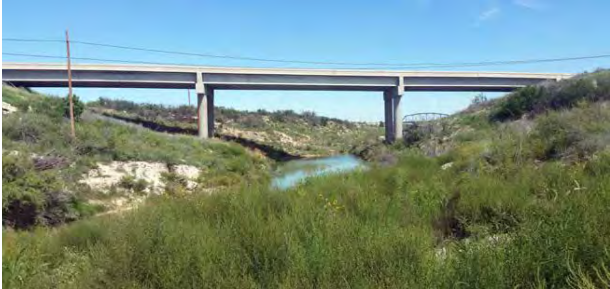
Figure 15. Delaware River bridge
